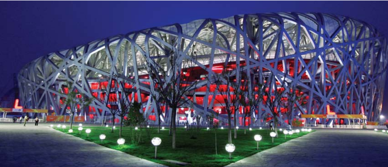
Beijing National Stadium (Bird's Nest) - GE's Showbiz CSR Discharge Lighting opened the dramatic Olympic Ceremonies
